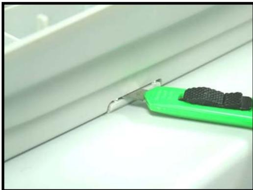
3. Use a cutter to break off the left tab of the side lid of the cable entry to power supply unit.
